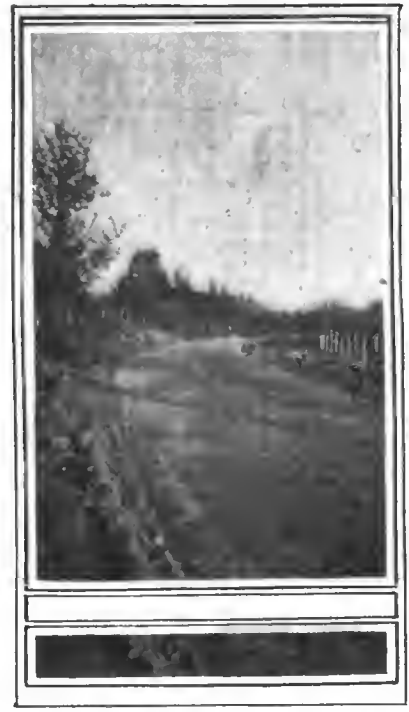
Completed Road Around the Ladder,
